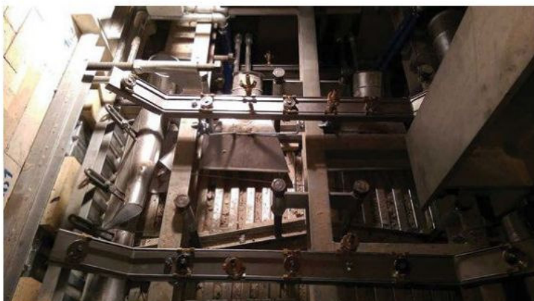
Throat with water registers and spray cooling during installation.
